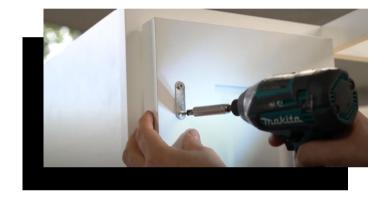
11. Repeat steps 9 - 10 for the bottom magnet pieces. Finish by adding on rubber door stoppers to the outer back corners of the door.
