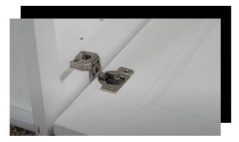
Door Adjustment Tip: \*\*If you notice a gap or miss alignment after screwing on the door, you can re-adjust the screws using a screwdriver in order to level and align your door. Be sure that a screwdriver, and not a drill, is used for adjustments since the hinge hardware is really delicate. The front screws adjust the door left and right, and the two side screws adjust the door to move up and down, and inward or outward.
