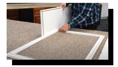
Assembly Tip: \*\*If the panels are not sliding into the dado
