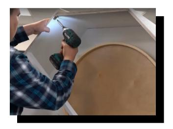
11. Further secure the corners of the cabinet frame by screwing on wooden brackets at each 90 degree corner.12. Further secure the back panel by screwing on the included, beveled plywood inserts along the pre-drilled holes.
