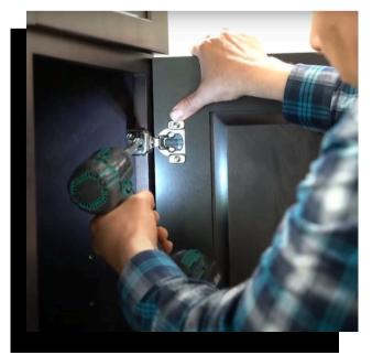
Door Adjustment Tip: \*\*If you notice a gap or miss alignment after screwing on the door, you can readjust the screws using a screwdriver in order to level and align your door. Be sure that a screwdriver, and not a drill, is used for adjustments since the hinge hardware is really delicate. The front screws adjust the door left and right, and the two side screws adjust the door to move up and down, and inward or outward.
