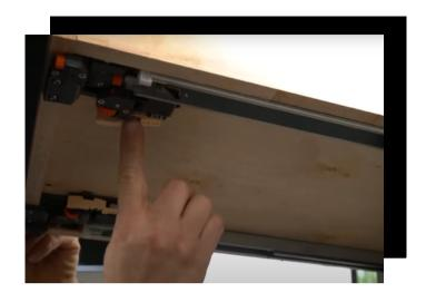
17. Align the flat side of the door hinges to the cabinet frame's pre-drilled hinge pin holes and screw in place. For finishing touches, stick on the rubber door stoppers to the outer corners at the back of the door and add in shelf pins and shelves (if applicable) to complete.
