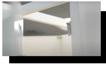
17. Next, stick the thin metal piece with a screw through one of the holes onto the magnetic white piece on the frame. Press the door lightly into the screw to create an indent on the door to map out where to screw in the metal bit. Before screwing on, double check that the screw length isn't too long, so that it won't run through the door.
